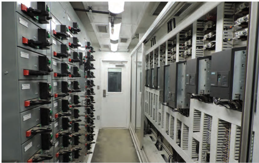
The inside of Carmen’s new modern control room with updated digital drives.
