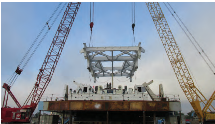
A two-crane lift setting the modified superstructure on the machine.
