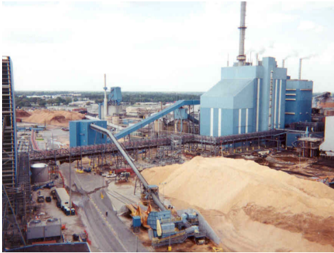
Wood Chip Conveyor Installation
