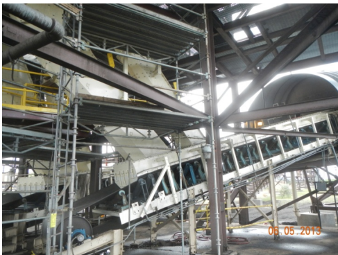
New Parallel Conveyors Replacing Troublesome Crossover Conveyors in Coal Transfer House
