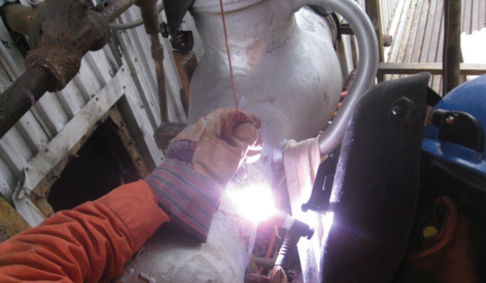
REPLACING AN 850 PSI STEAM VALVE
